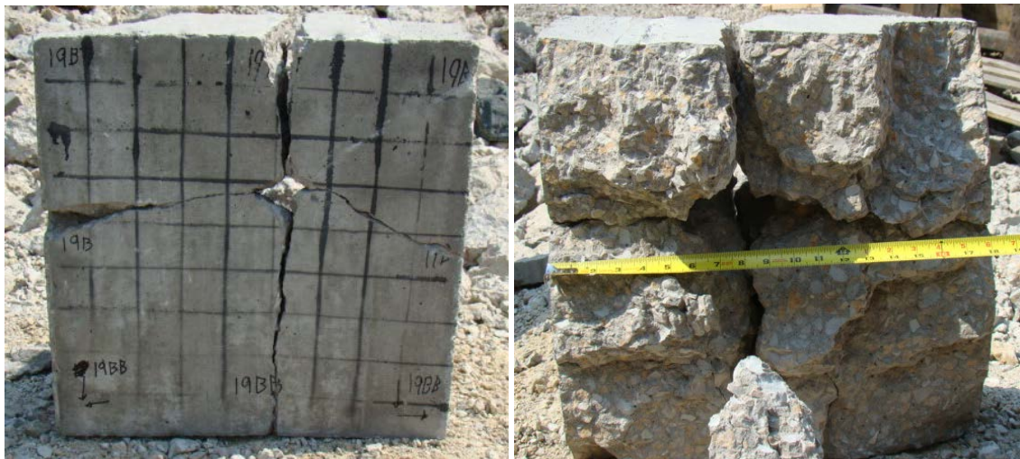
Figure 4.24: Block 19, back face and interior views after impact
